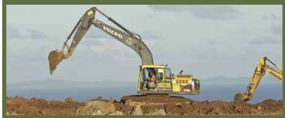
Mine Pit Development at Cagdianao Mine Site
