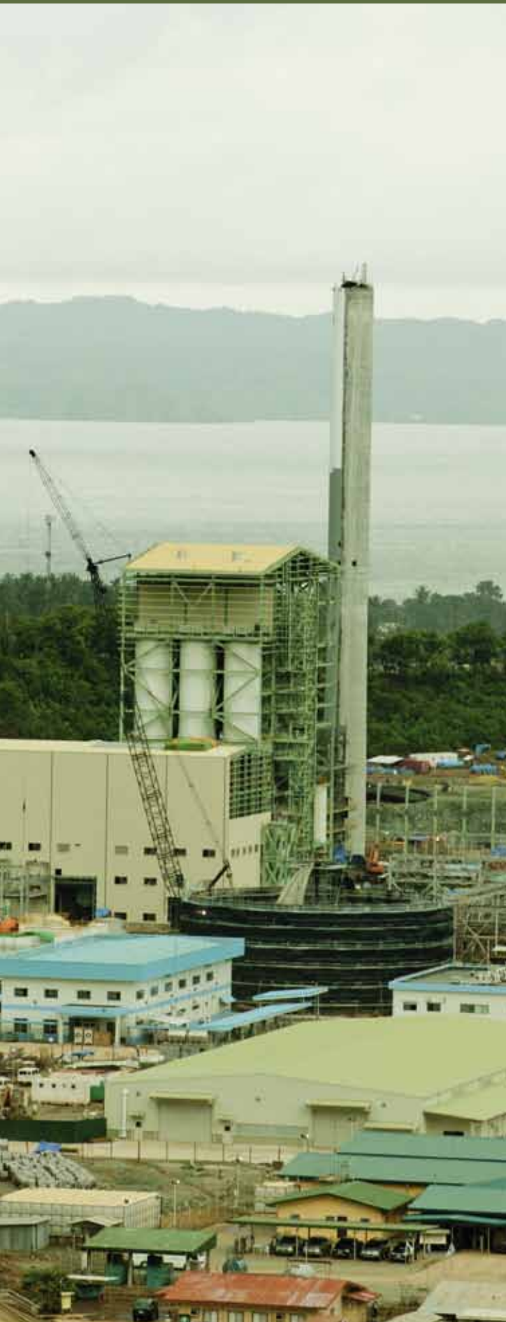
Taganito HPAL Plant Project Construction
