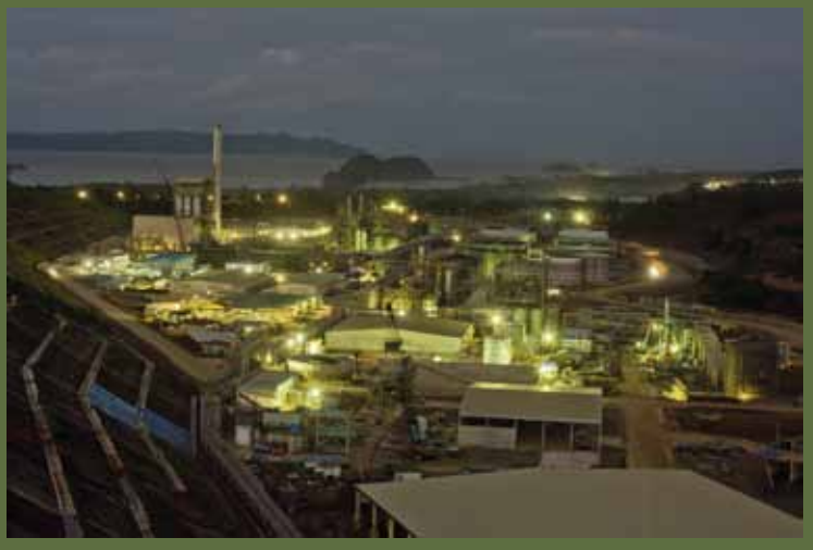
Taganito HPAL Plant Project Construction
